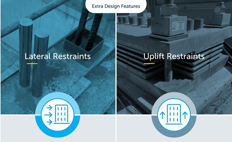
In situations where lateral loads are present (such as wind, etc.), consideration should be given to the lateral restraint of the building.
