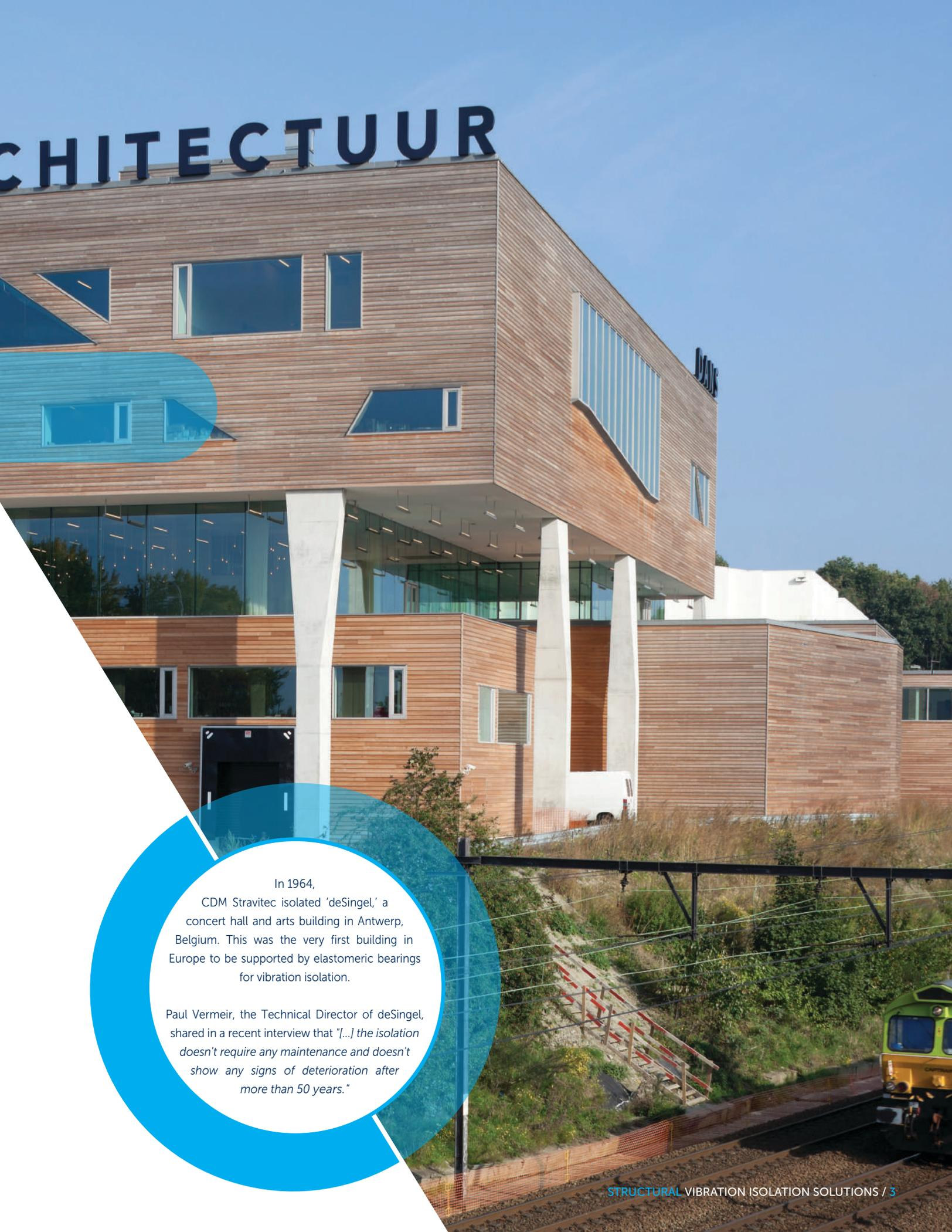
In 1964, CDM Stravitec isolated 'deSingel,' a concert hall and arts building in Antwerp, Belgium. This was the very first building in Europe to be supported by elastomeric bearings for vibration isolation.
